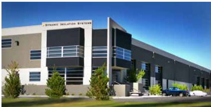
Dynamic Isolation Systems design and manufacturing facility in Nevada.
