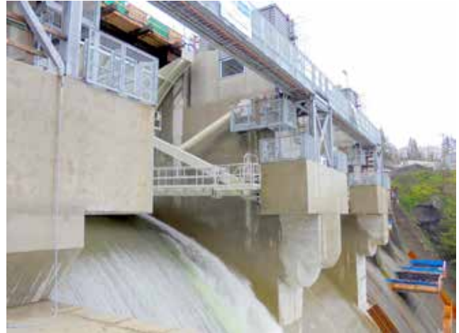
Canada's Ruskin Dam used 3D isolation to protect mission-critical equipment.
